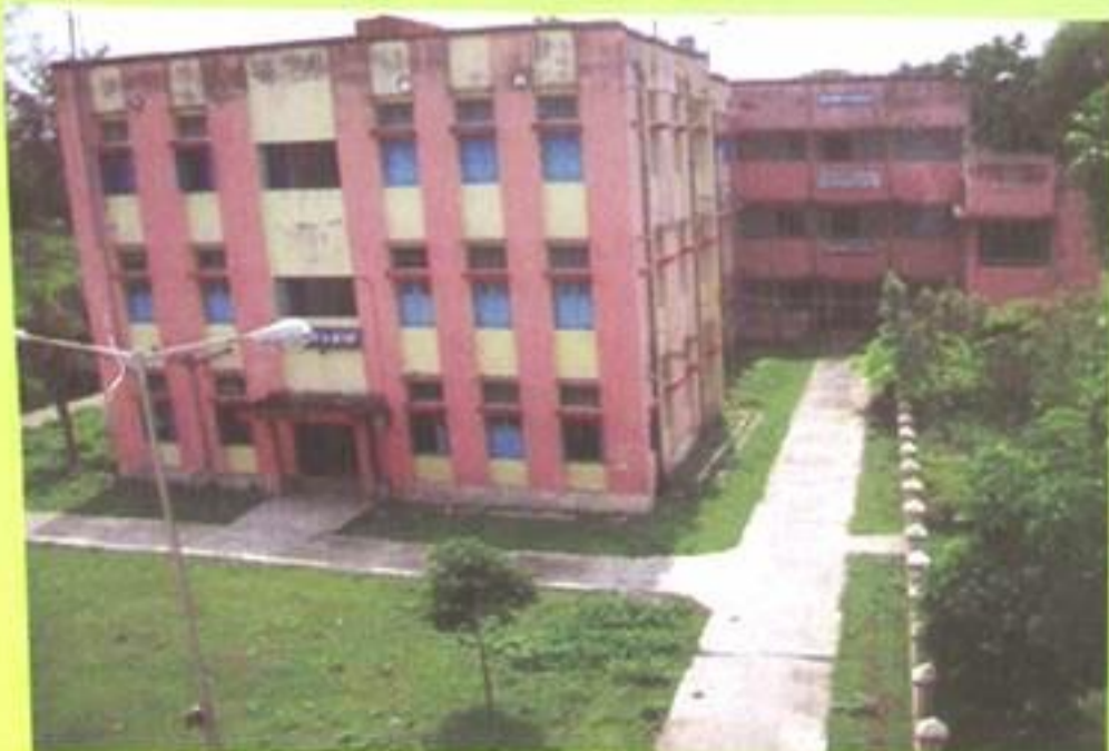
Biological Science Building
